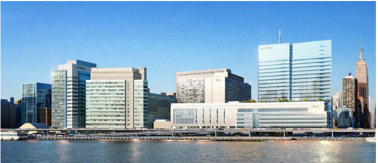
Figure 2.5b NYU Langone as seen from the East River, 2018. The Energy Plant is the foreground lower building in the middle of the image. Source: NYU Langone
